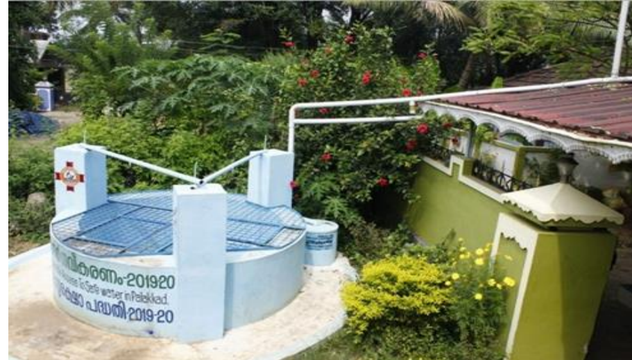
New storage wells and connecting with roof and surface rainwater
