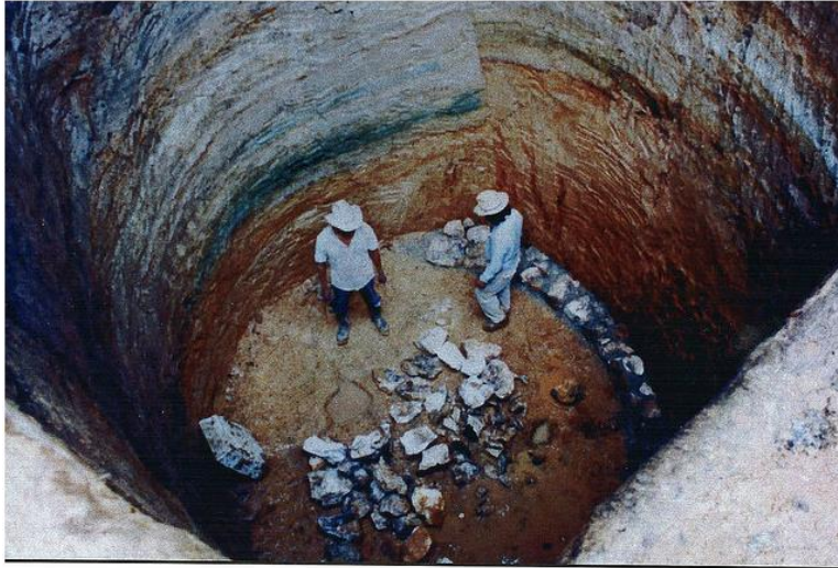
Refurbishment or deepening of existing dug wells
